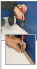
piece of panel fixing extrusion and place on the line previously drawn. Drill and fix the panel fixing extrusion to the back of the tray using the pre-drilled holes in the extrusion. The extrusion will be approximately
