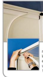
STEP 11 Insert the rubber gasket into the underside of the roof and also clip the roof capping into the exposed underside of the roof.
