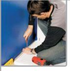
Take one of the side pieces of panel fixing extrusion and place on the line previously drawn along the side of the tray, making sure that the holes
