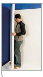
Locate the side panel into the back panel, turn and clip into place as shown in the picture.
